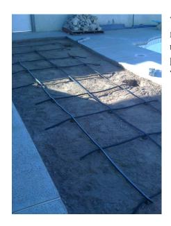
Waste steel-belted reinforced tire cable used for concrete patio reinforcement which replaces rebar.
